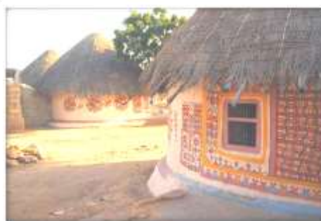
Figure 4, Exterior walls circular Adobes
